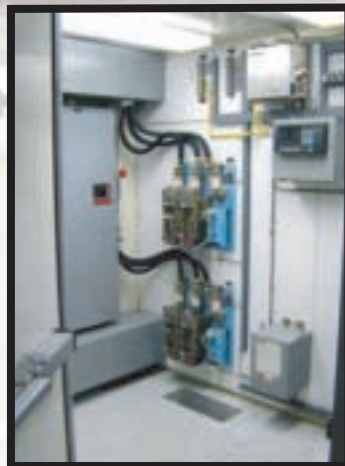
Detail: Switches, SCR Units
