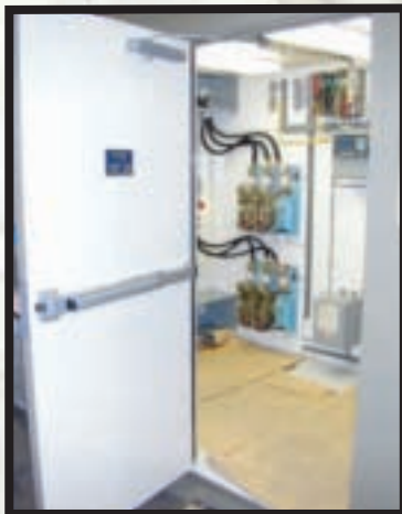
Heater Control Building
